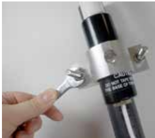
Figure 14. Mast Mount Antenna – Tighten nut on mounting bracket
